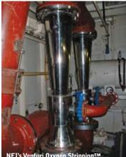
NEI's Venturi Oxygen Stripping™ ballast water treatment system.
